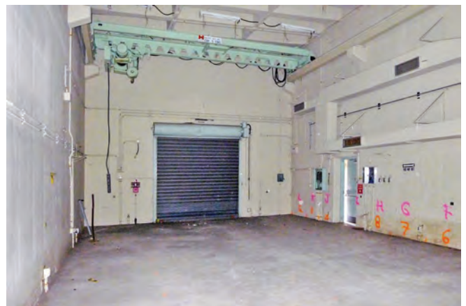
MSR warhead handling building interior showing main door and overhead gantry crane
